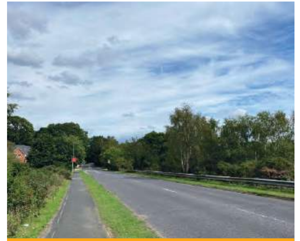
Arrival into Hedge End along St Johns Road beyond the M27 bridge enhanced by mature tree belts and woodland that help to conceal the settlement edge.
