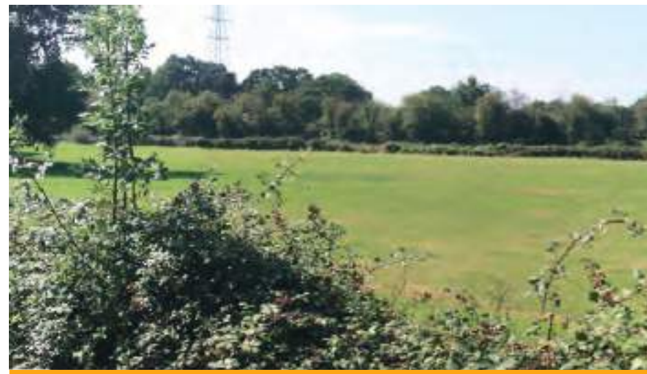
View across Sub Area I 1 showing open farmland in Boorley Green with field boundary and railway vegetation preventing views to Hedge End.
