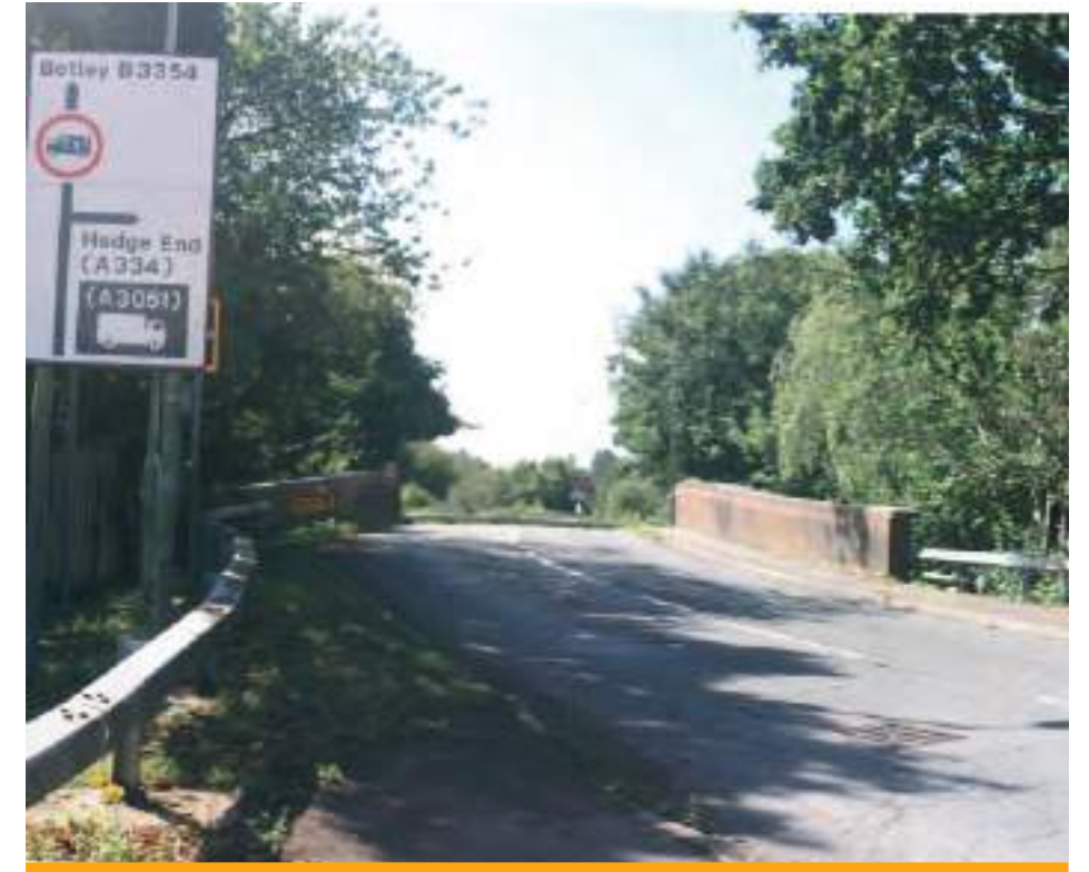
View from railway bridge and surrounding vegetation defines the junction of the three settlements.
