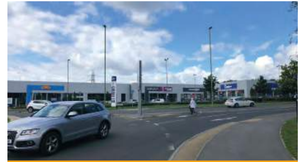
Typical view of Hedge End Retail Park.
