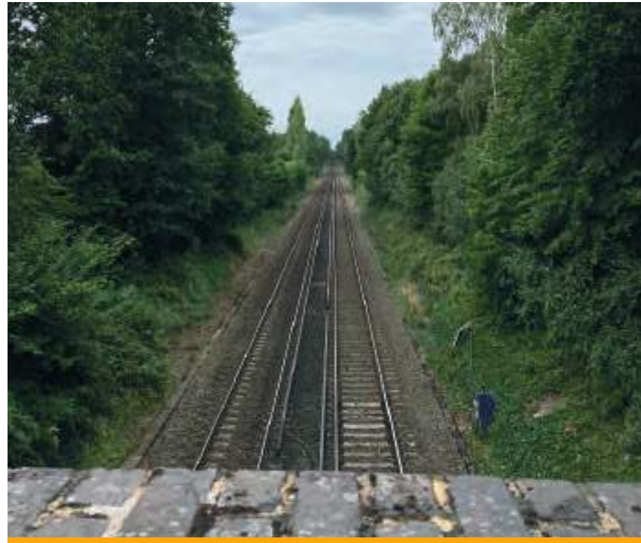
Typical view of railway line with vegetated slopes / embankments forming strong sense of enclosure.
