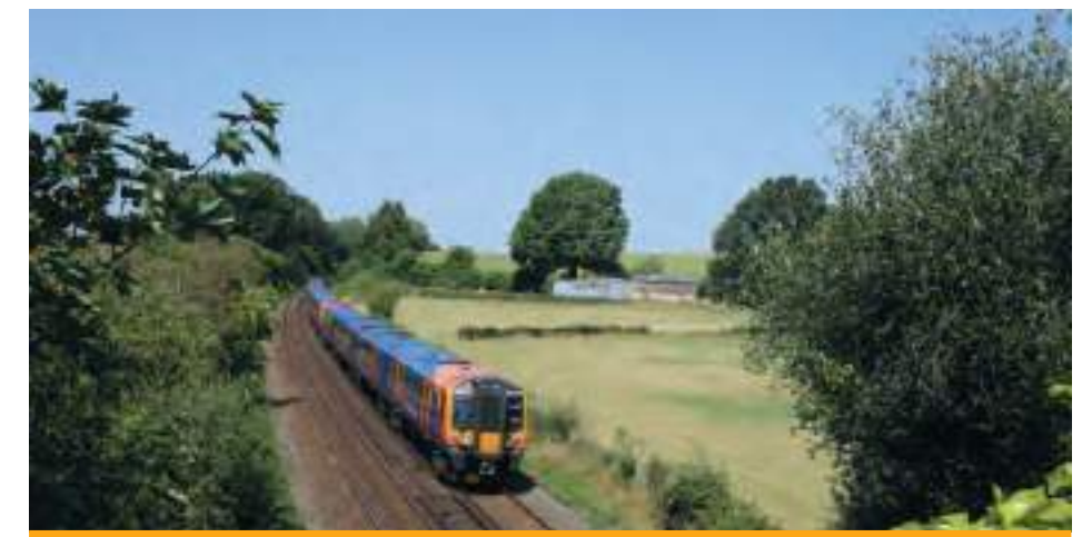
View from railway bridge overlooking the sunken railway Line and vegetated embankment looking towards Boorley Green.
