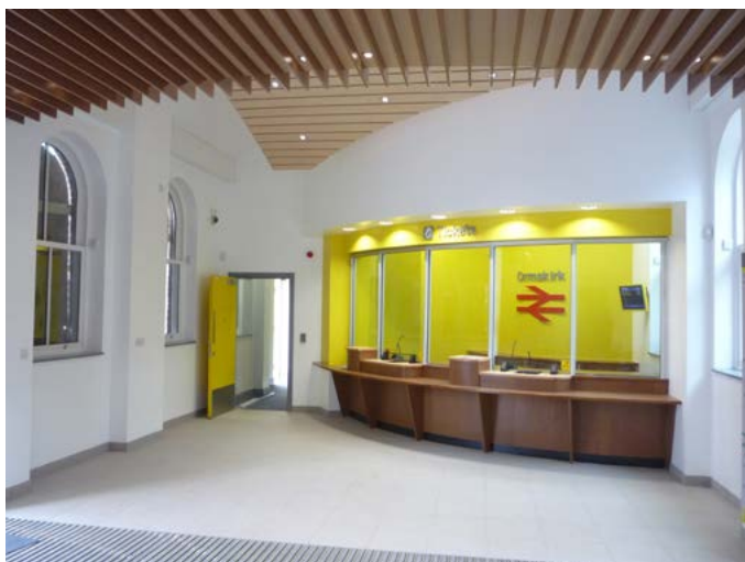
Ormskirk station redevelopment. This project was funded by: Lancashire County Council, Merseytravel, Railway Heritage Trust, West Lancashire Borough Council, Northwest Regional Development Agency (NWDA) and National Stations Improvement Programme
