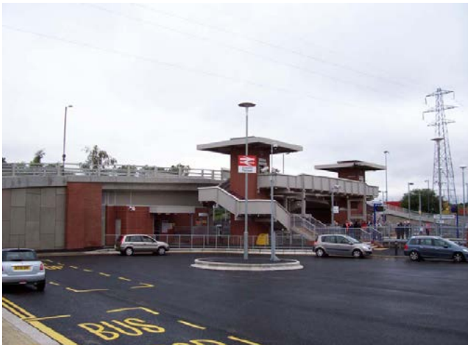
Coleshill Parkway new station (Funded by: Laing Rail, DfT through LTP, Warwickshire County Council and North Warwickshire District Council)
