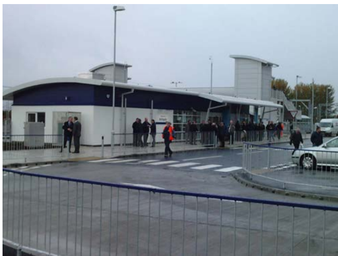
Bathgate - new station (Funded by: Transport Scotland)
