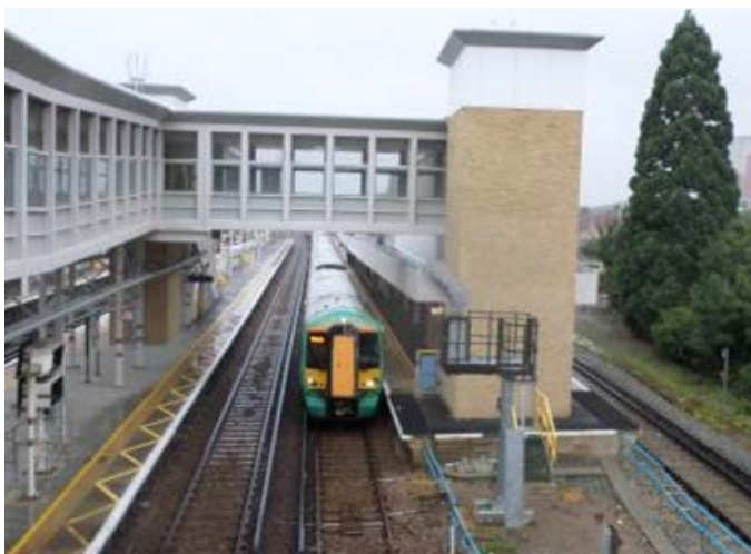
New Cross Gate Station, Access for All fund
