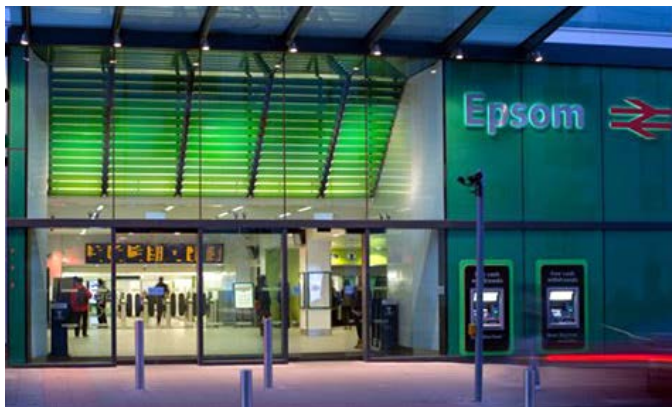
Epsom station redevelopment (Funded by: Network Rail and Kier Property)
