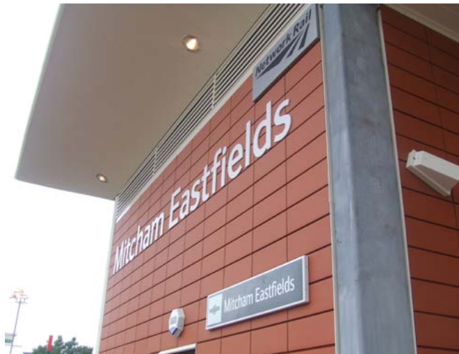
Mitcham Eastfields - new station (Funded by: Network Rail)
