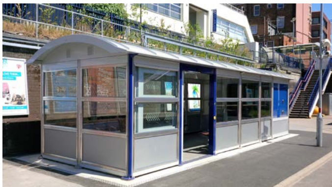
West Hampstead station following completion of a National Stations Improvement Programme project: waiting room and customer service facility.
