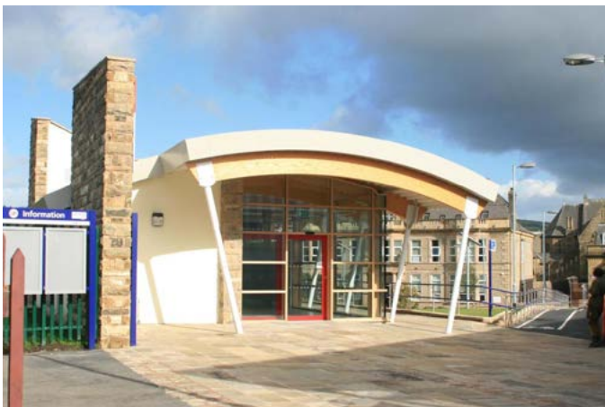
Accrington eco-station redevelopment (Funded by: Lancashire County Council, Hyndburn Borough Council, National Stations Improvement Programme and European Regional Development Funding)
