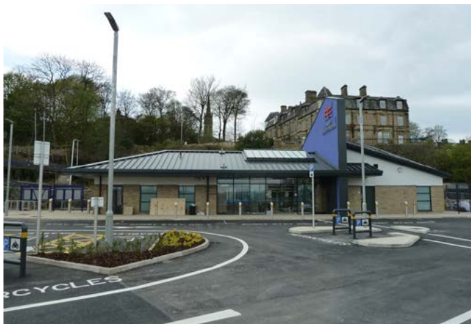
Burnley Manchester Road - redeveloped station (funded by Burnley Council, Lancashire County Council and European Regional Development fund)
