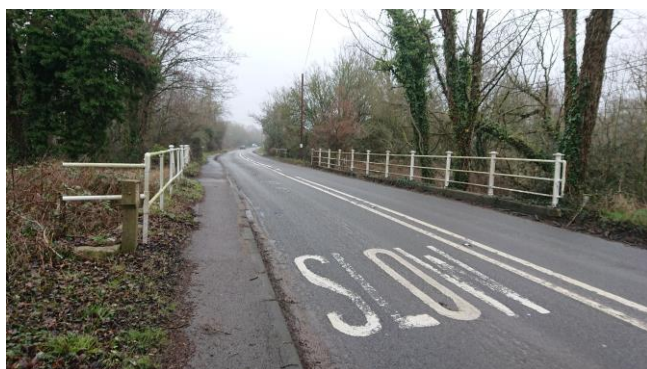
Photograph 3: Footway South of River Itchen Bridge
