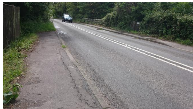
Photograph 4: Footway North of River Itchen Bridge
