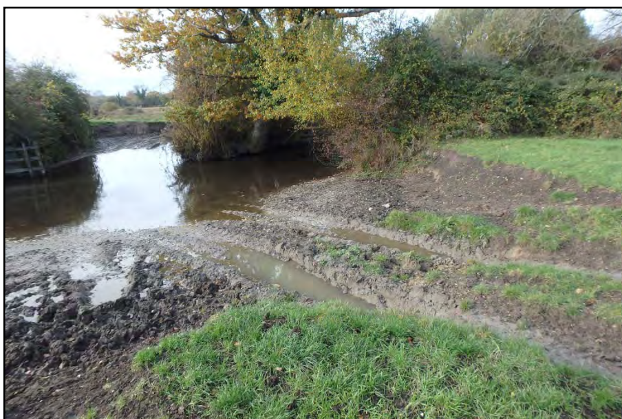
Photograph 2: Ford at the junction of watercourses 10 and 13 used for cattle and vehicular crossing
