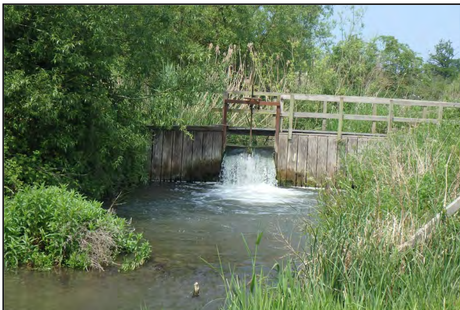
Photograph 1: Main control structure near the centre of the site
