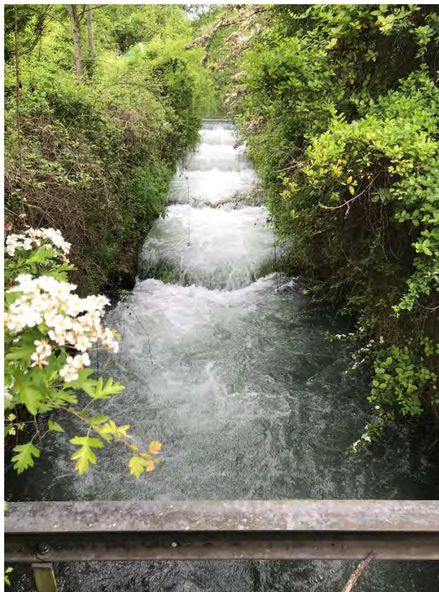
Figure 6.16: Cascade upstream of the bridge at Highbridge
