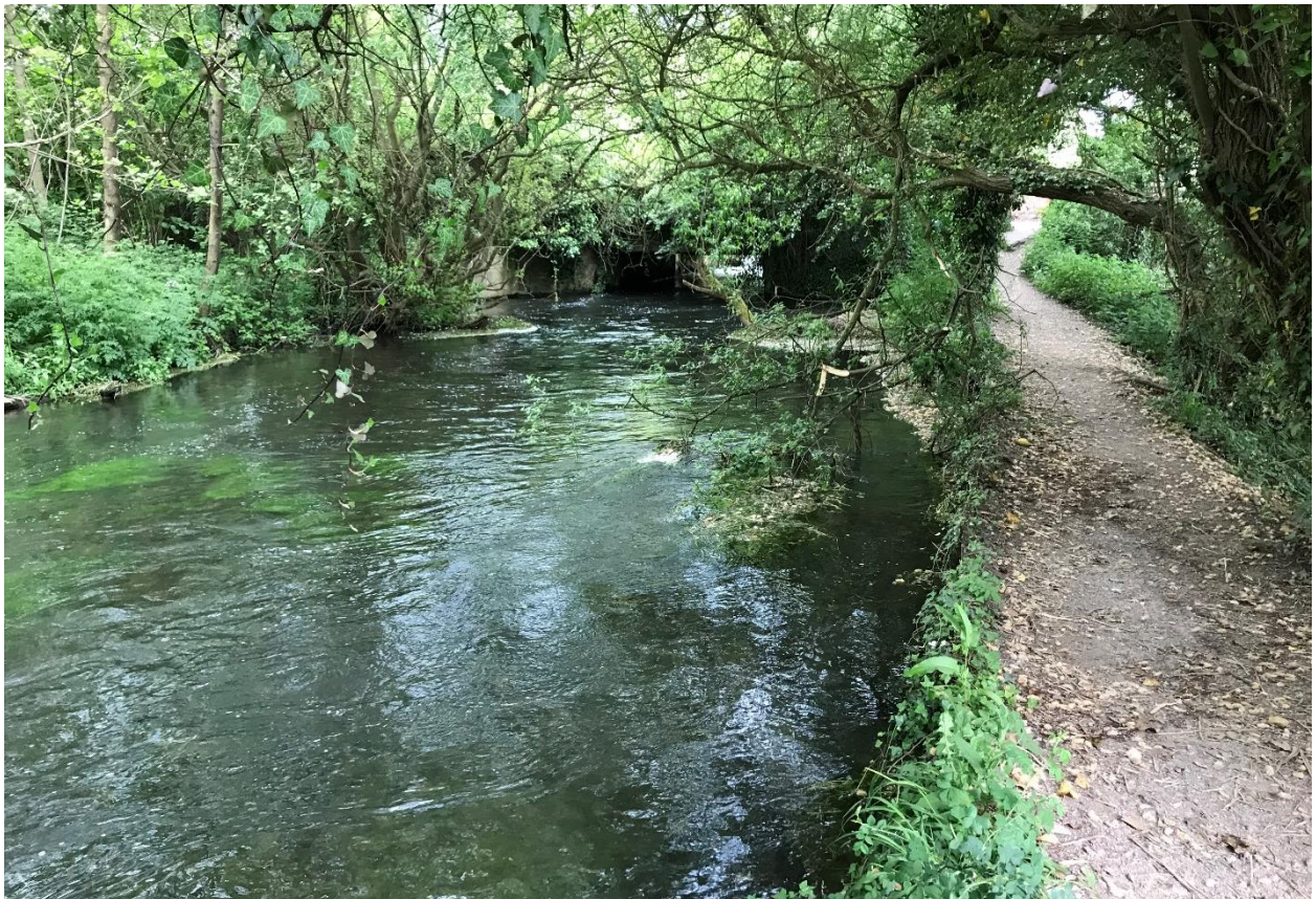
Figure 6.18: Itchen Navigation downstream of the bridge at Highbridge looking upstream under the bridge from east bank. Note the absence of marginal and emergent vegetation
