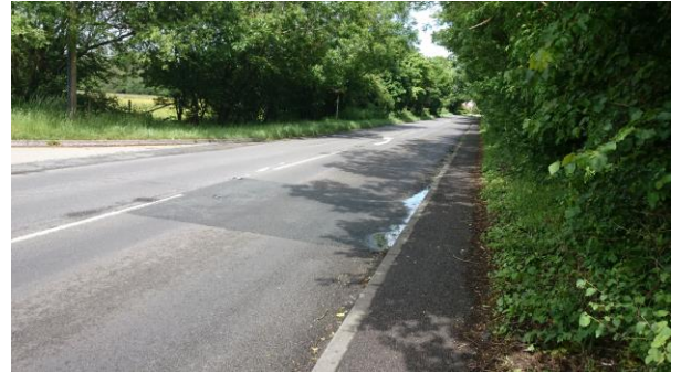
Photograph 6: Highbridge Road Frontage
