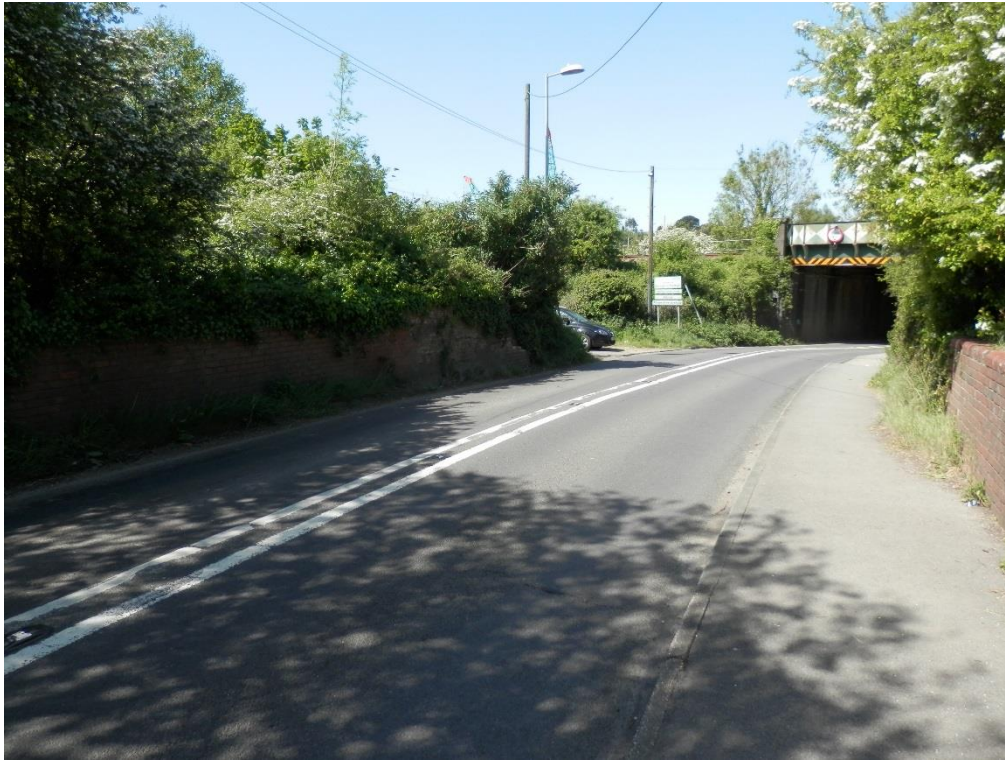
Photograph 1 Looking west over the top of the bridge
