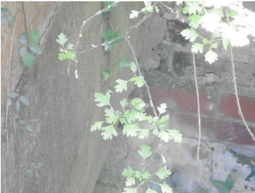
Photograph 9 Brickwork abutment at the North west corner of the bridge
