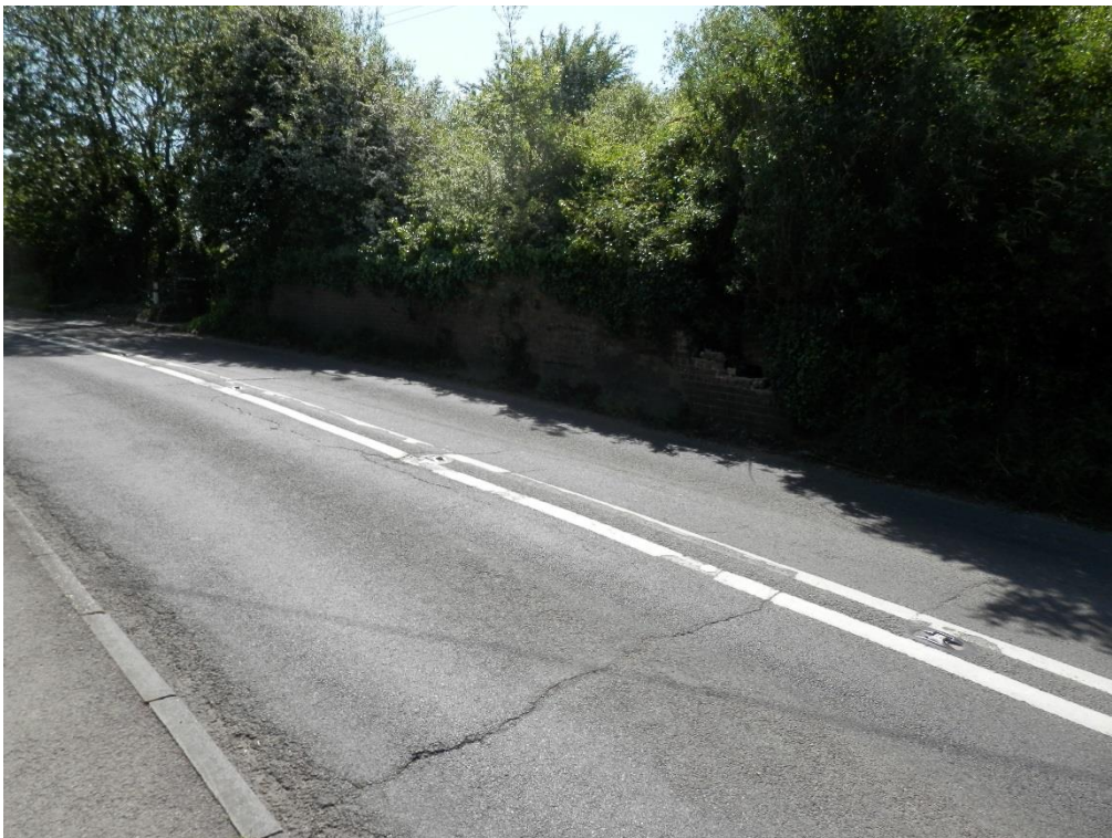
Photograph 2 Looking south east over the top of the bridge
