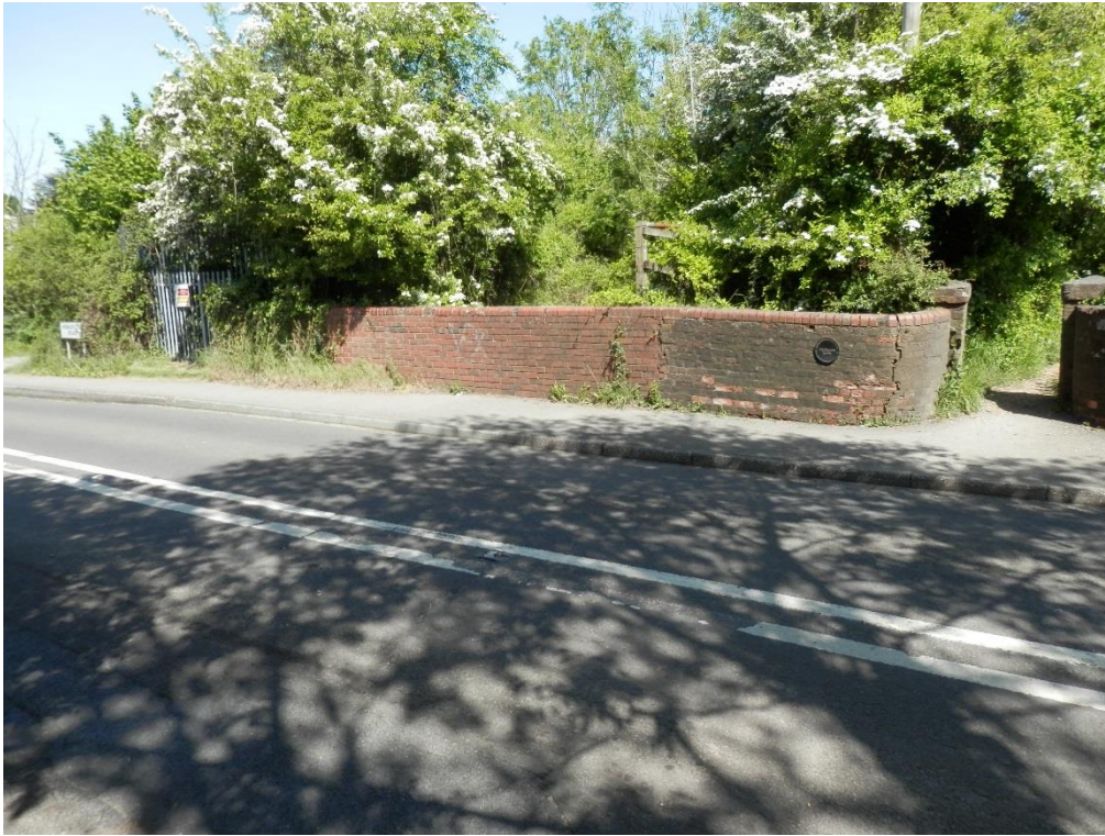
Photograph 3 Looking north over the top of the bridge
