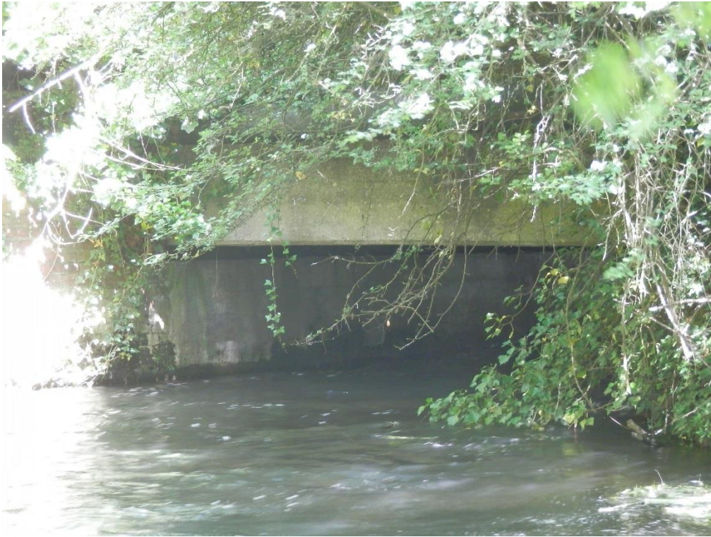
Photograph 5 View of the South elevation of the bridge
