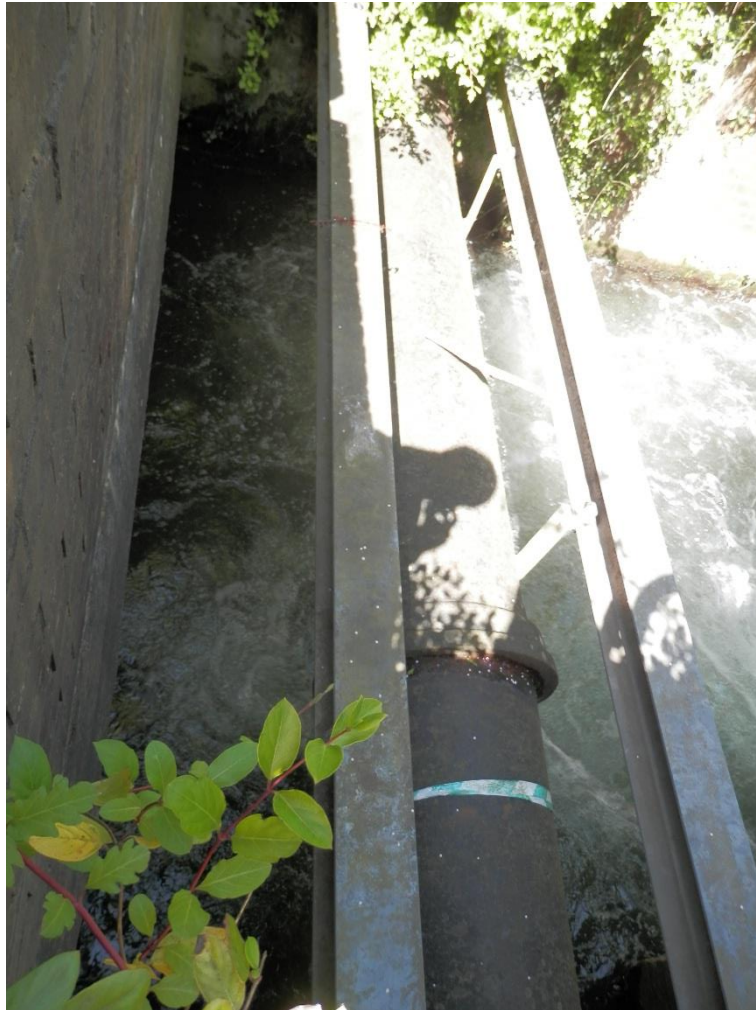
Photograph 10 Pipe bridge to the North of the existing bridge
