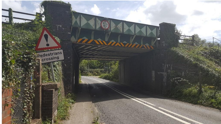
Photograph 6: Western Approach to Railway Bridge
