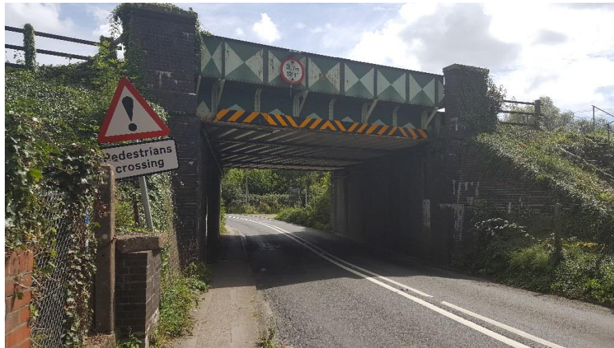
Photograph 5: Conditions under Allbrook Railway Bridge (view from the West)
