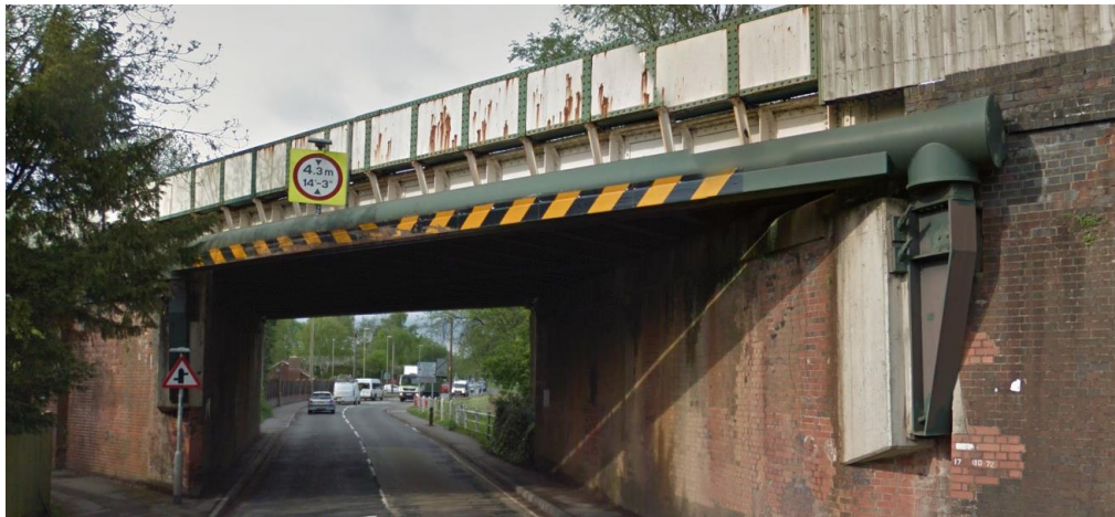
Photograph 9: Protective beam at Greatbridge Road, Romsey
