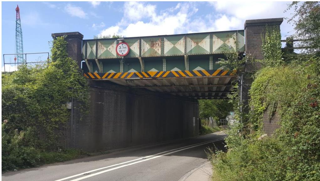
Photograph 7: Eastern Approach to Railway Bridge
