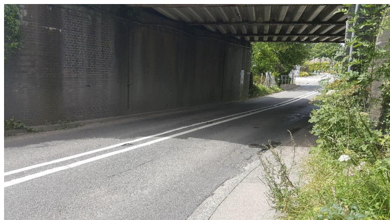
Photograph 4: Conditions under Allbrook Railway Bridge (view from the East)
