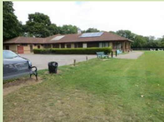
Well-maintained benches at Norman Rodaway Pavilion
