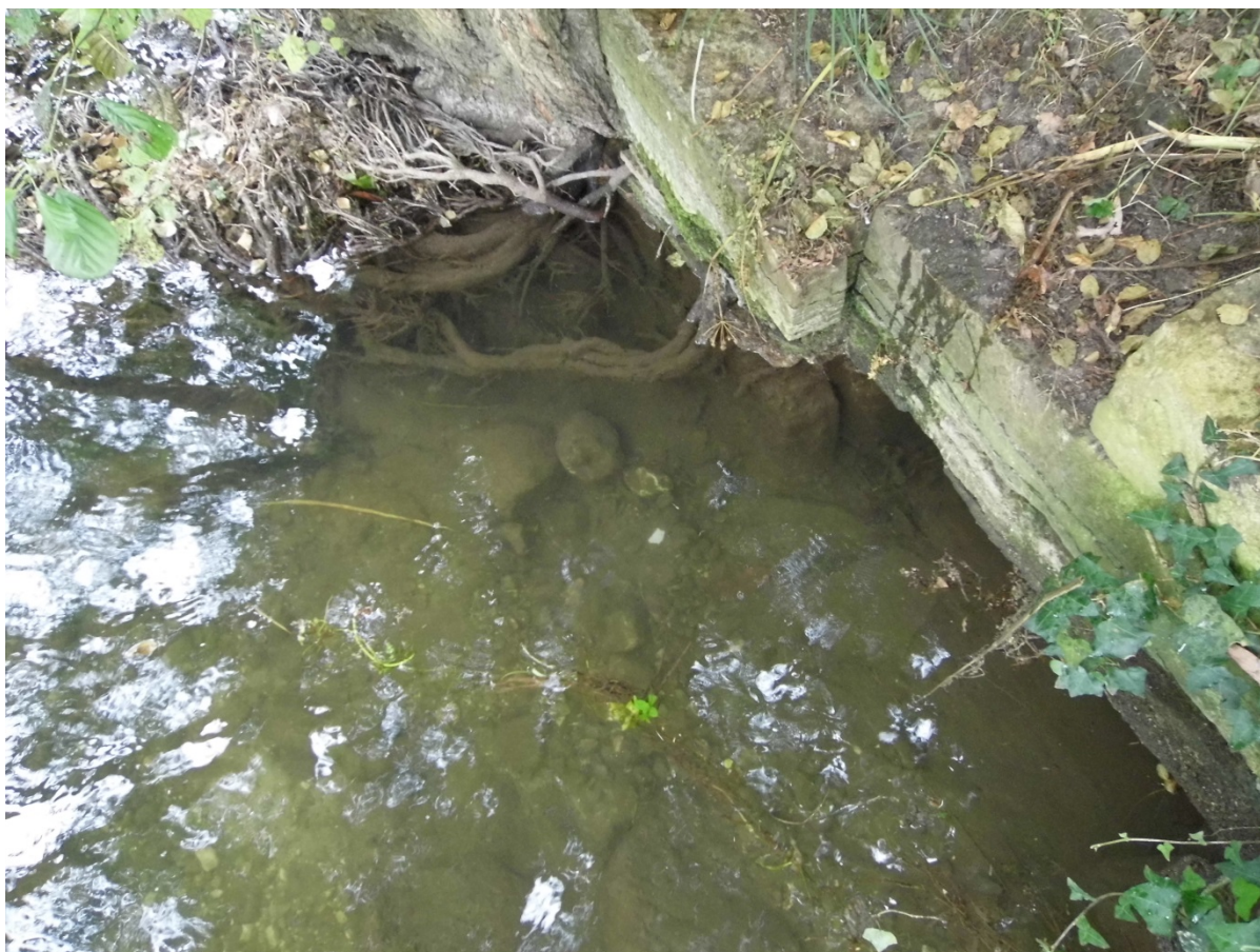
Figure 6: Existing offtake structure associated with the Itchen Navigation.
