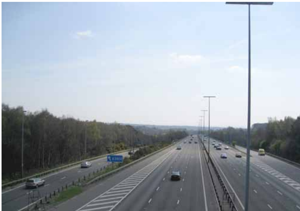
Figure 30. M27 motorway near Netley Hill
