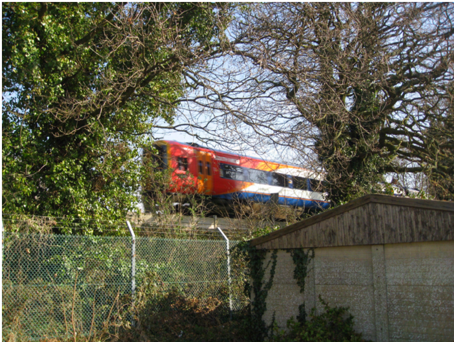
The railway embankment seen from the site
