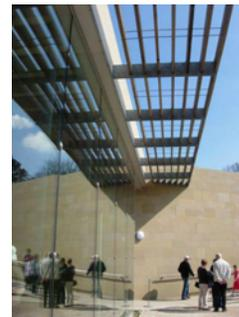
Fig 3.6 brise soleil solar shading
