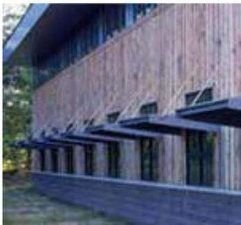
Fig 3.2 Light Shelves (Light bounces off the top of the light shelf into the ceiling of the first floor offices. The overhang shades the window below it).
