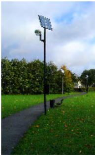
**Solar Street Light:** The Solartech “Pathfinder” street light. The compact fluorescent lamp is powered by a 110W solar panel. In summer this unit stays illuminated all night long. In winter the light is dimmed by 50% and shines for at least 3 to 6 hours. Although this performance would not be suitable for illuminating the highway, it is suitable for other applications and the technology is improving very rapidly.
