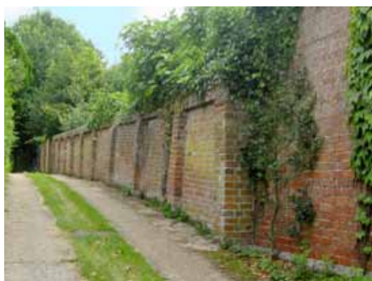
Listed wall bounding The Old Rectory
