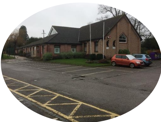
Fig 7: The Botley Centre parking area
