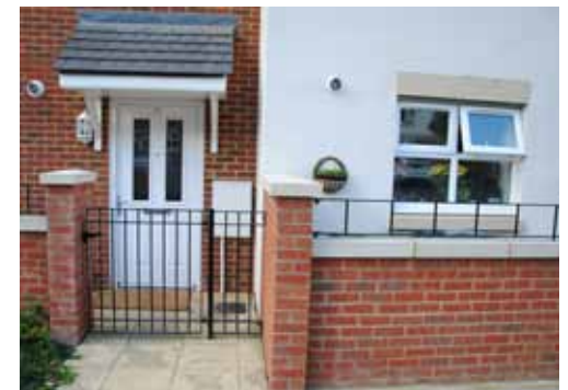
Fig 33. Attractive and robust front boundary structures screening wheelie bins at Bodmin Road, Bishopstoke
