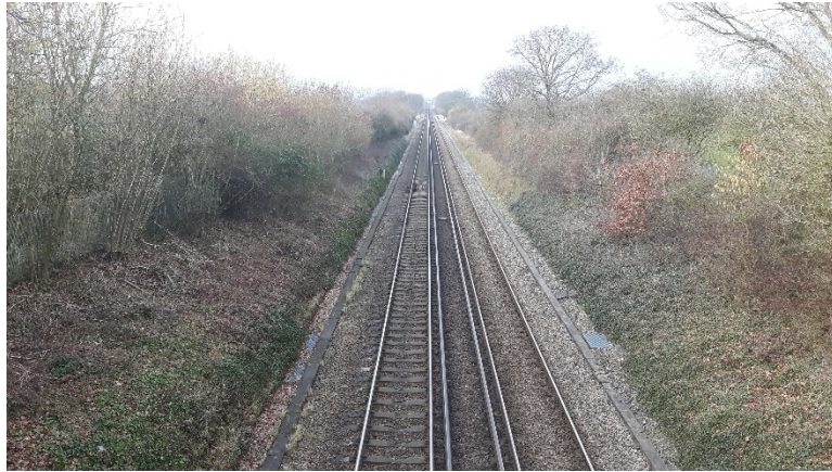
View from Allington Lane road bridge looking towards Eastleigh
